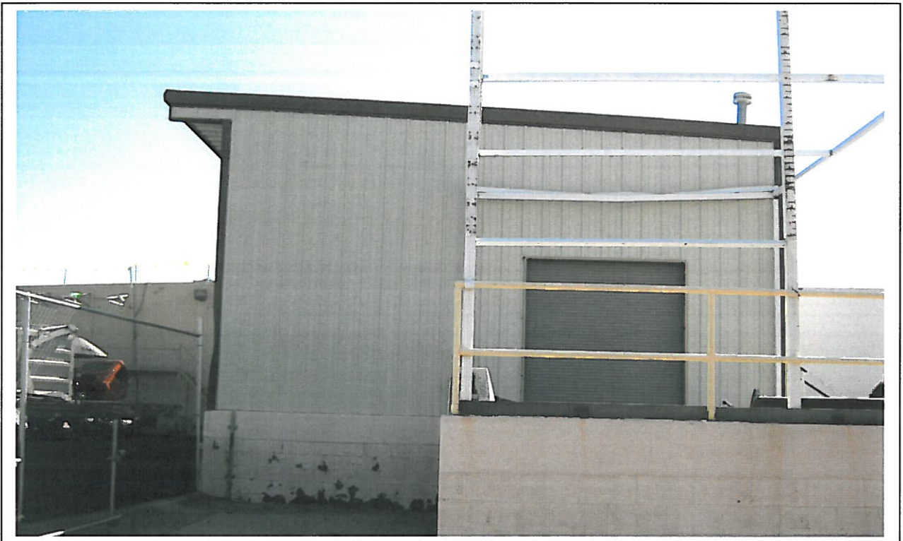
No. 2 – West Elevation of loading/unloading dock and enclosed storage building.
