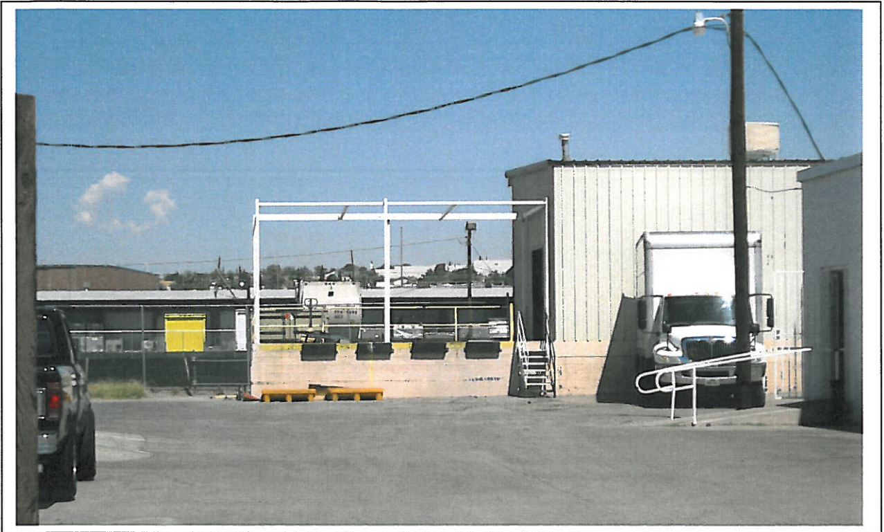
No. 1 – South Elevation of loading/unloading dock.
